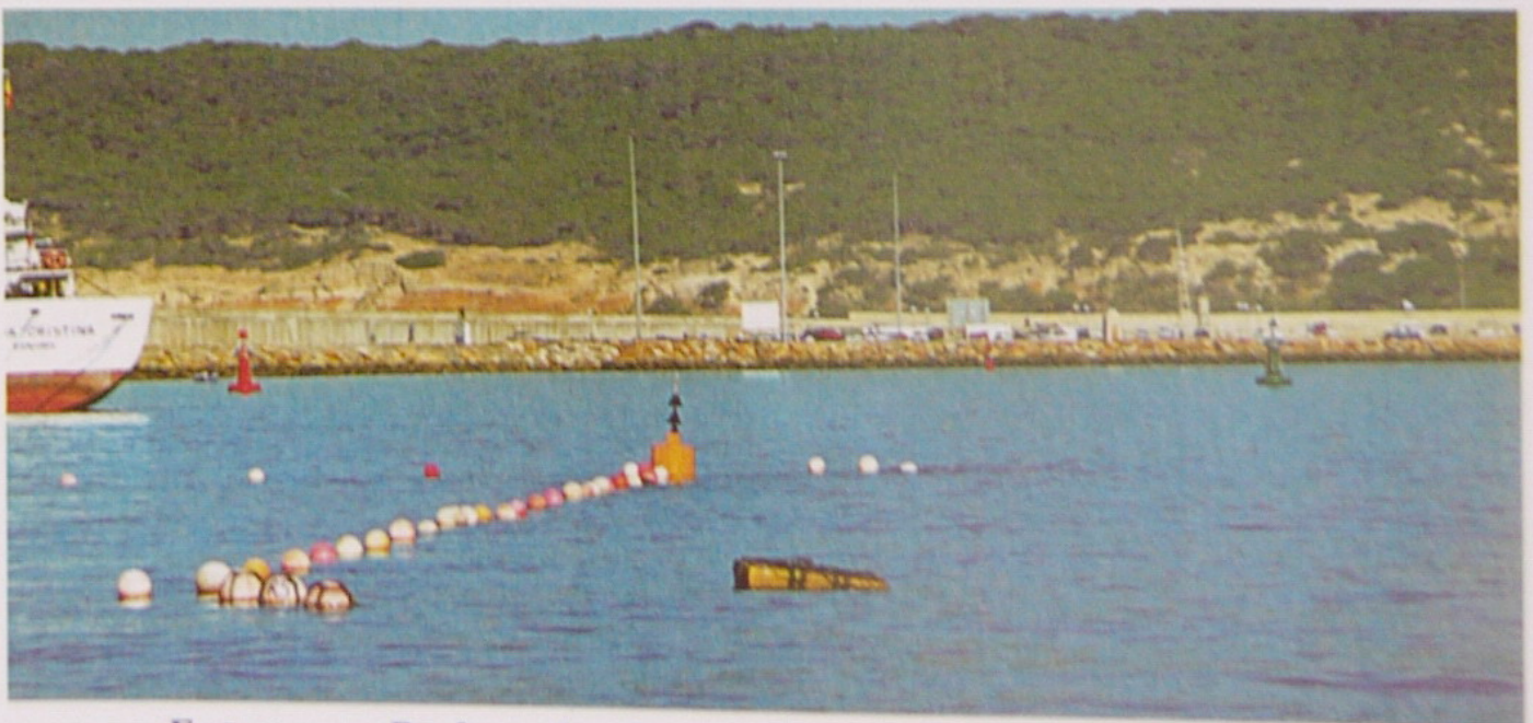
Entrance to Barbate showing north cardinal at inshore end of net
