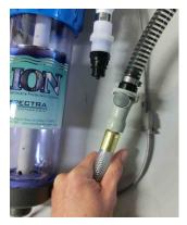
Removing hose to sea strainer from the "to strainer" pigtail.
