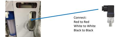
If a 2nd Tank Level Sensor is going to be installed, it should be installed at the base of the second tank. If monitoring 2 water tanks, they must be isolated from each other with a valve to read properly.
