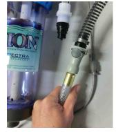
Removing hose to sea strainer from the "to strainer" pigtail.
