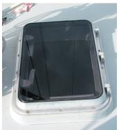
**How it works:** The acrylic is stuck with either bituminous mastic or double-sided foam filled tape on the horizontal surface (part on the aluminium frame and part on the rubber closing seal). Mastic is then used to fill the gap around the edge.
