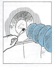
remove trapped air. Apply the second layer and wet it out. Squeegee. Repeat this process a layer at a time, mixing fresh epoxy as needed, until the repair is slightly below the surface.
