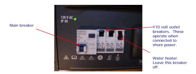
Island Beat is equipped with 2 110v outlets, one located by the 12 volt and 110 volt panel and one located in the galley. These will operate when the boat is connected to shore power or when you use the inverter. See next page for further details.
