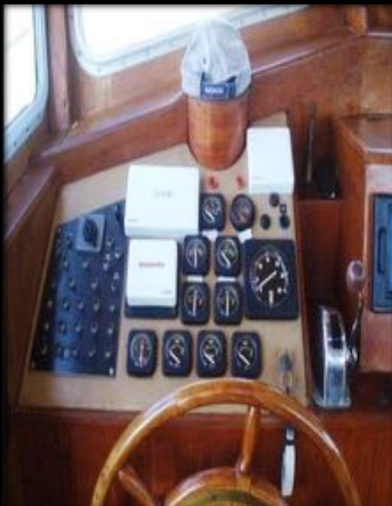
Typical Wheelhouse controls
